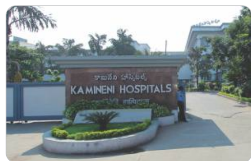
Kamineni Hospital, LB Nagar
